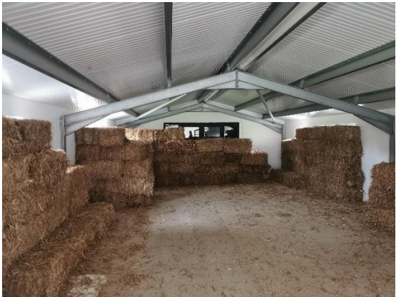
Hay storage on the mezzanine floor
